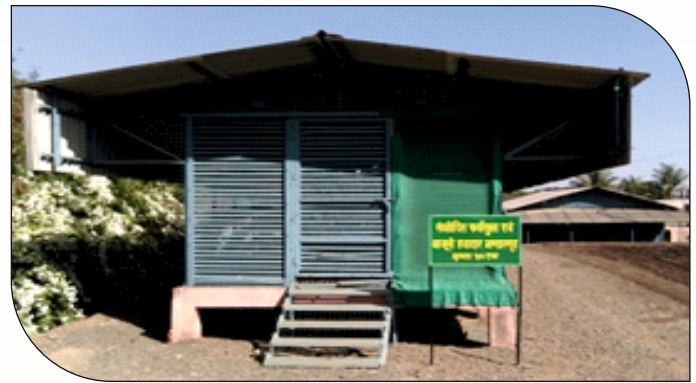
Fig 2. High volume storage (50 MT) structure
